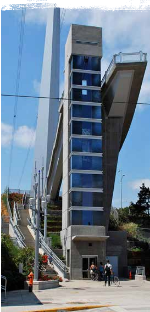
Gibbs Street Pedestrian Bridge, an example of an existing bridge elevator in Portland, Oregon
